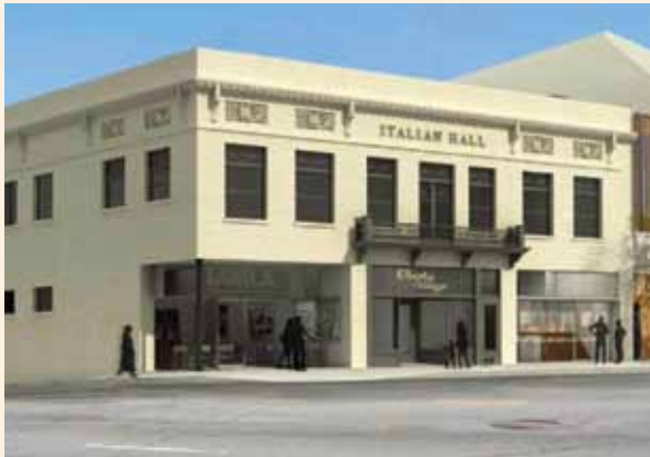
Exterior view of the IAMLA post-restoration
